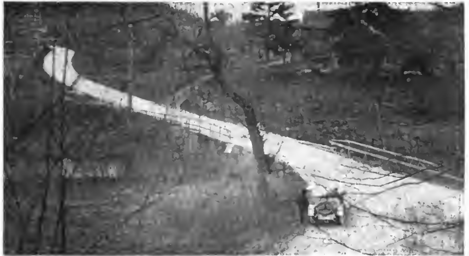
This, One of the Many Windings, Is Near Hawthorne.
